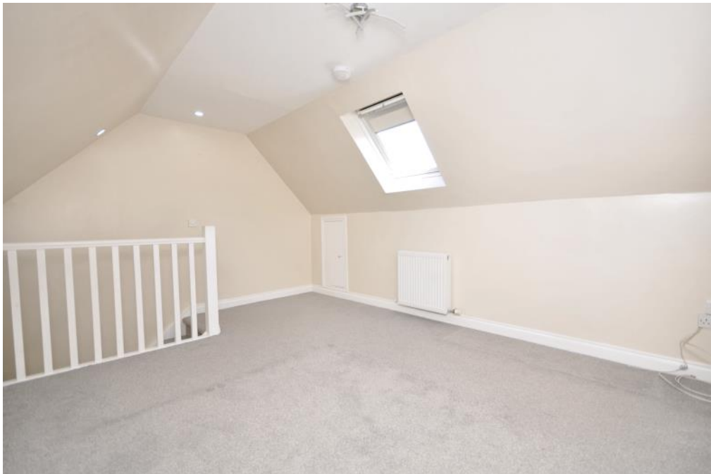
Floored & Lined Attic
