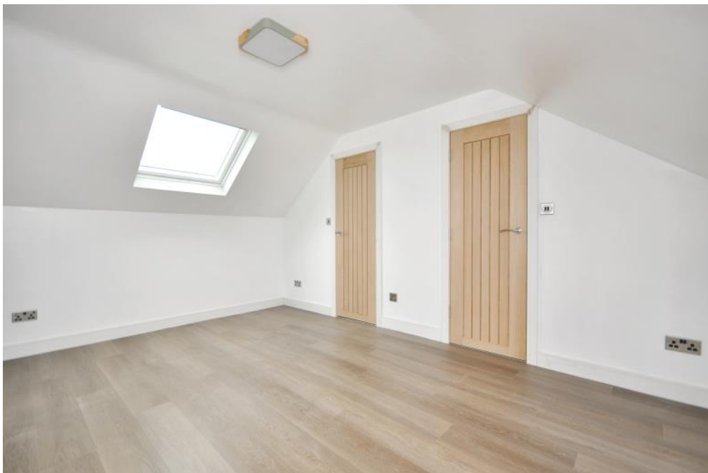
Floored and Lined Attic
