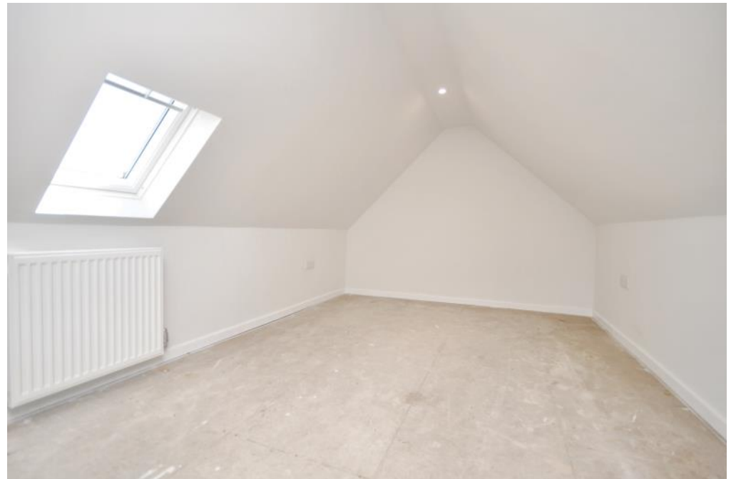
Floored & Lined Attic
