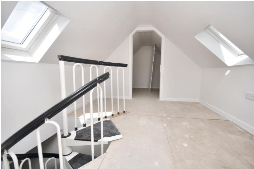
Floored & Lined Attic
