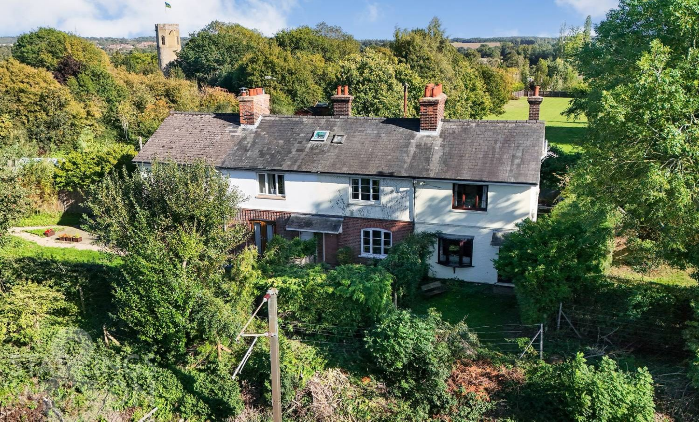
Station Cottages, Swainsthorpe - NR14 8PP
