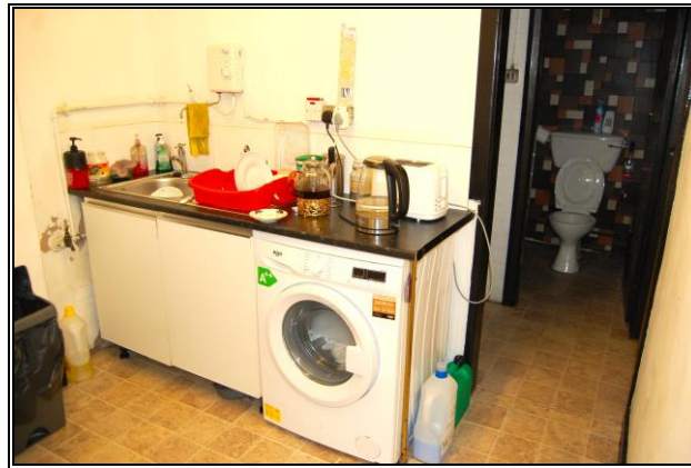
Basement, Kitchen & WC
