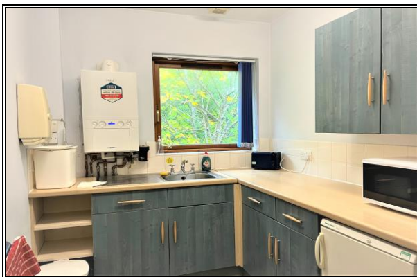
First Floor Kitchen
