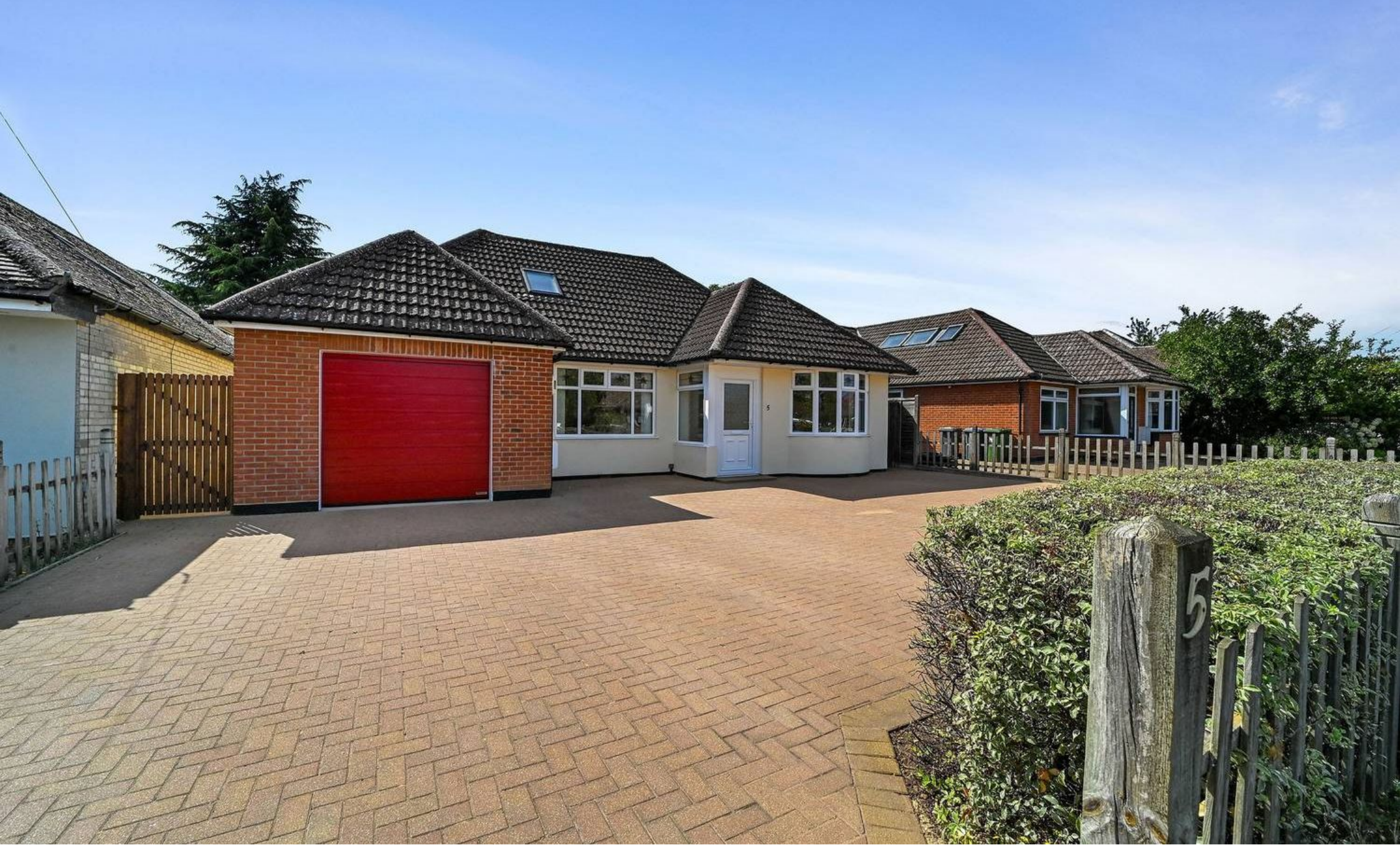
5 Black Tiles Lane, Martlesham Woodbridge
