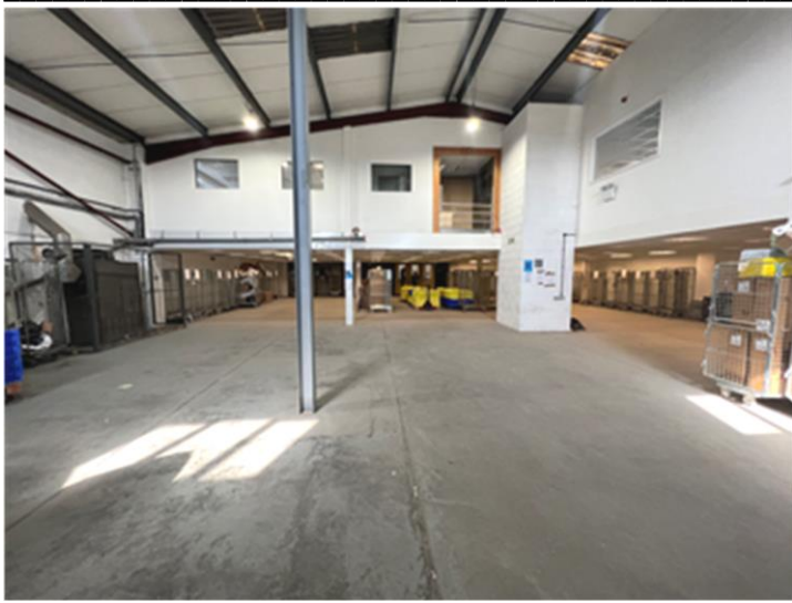
Ground Floor Warehouse
