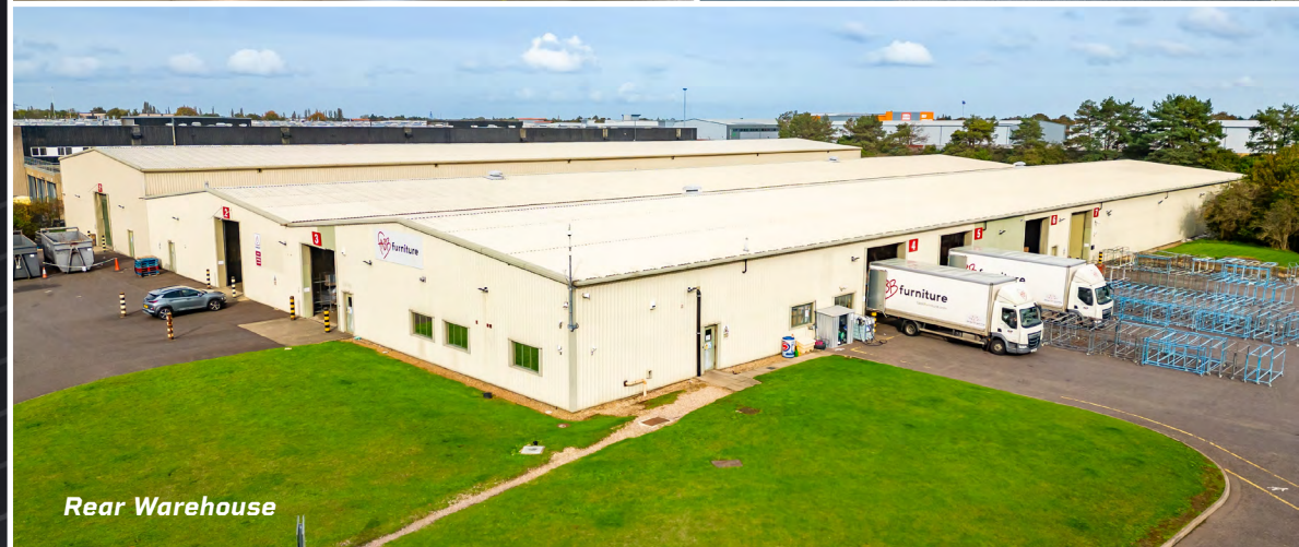
Rear Warehouse Offices
