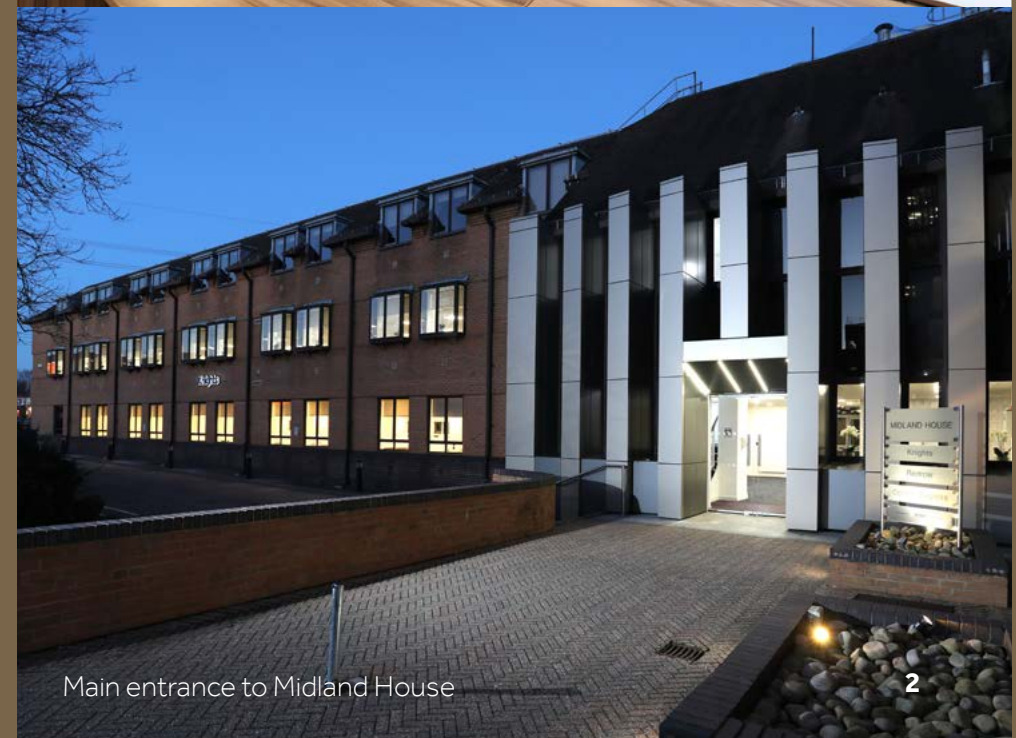
Ground floor office
