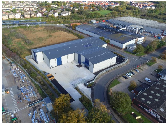
Note: Photographs taken in September 2020
