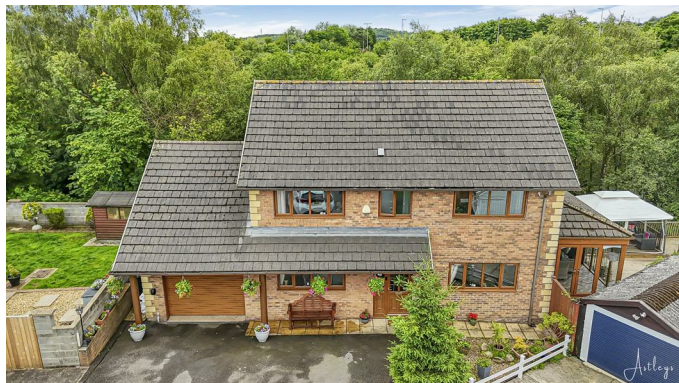
Front double glazed entrance door into:
