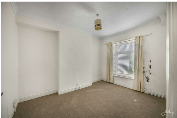
Window to rear, radiator, coving
