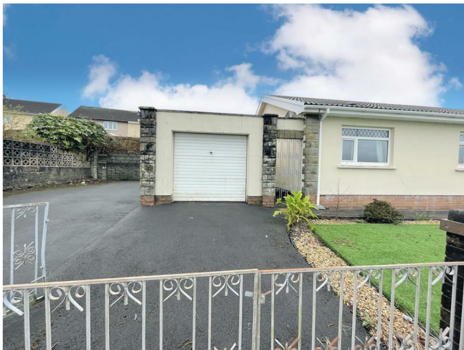
Single garage with up and over door.
