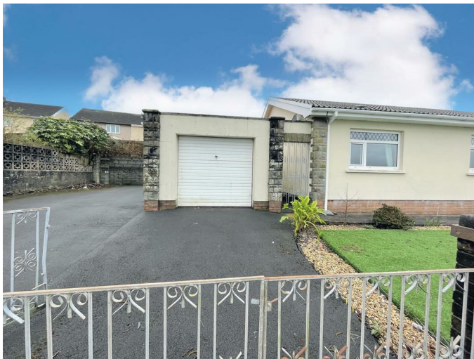
Single garage with up and over door.
