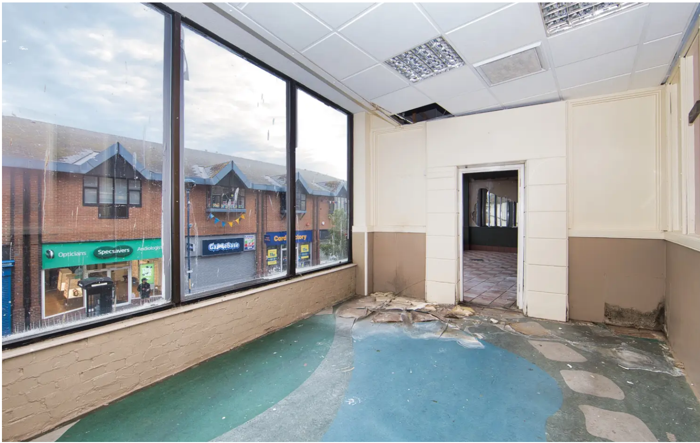
Ground Floor Sales Area 58' 9" x 32' 6" (17.90m x 9.90m)
