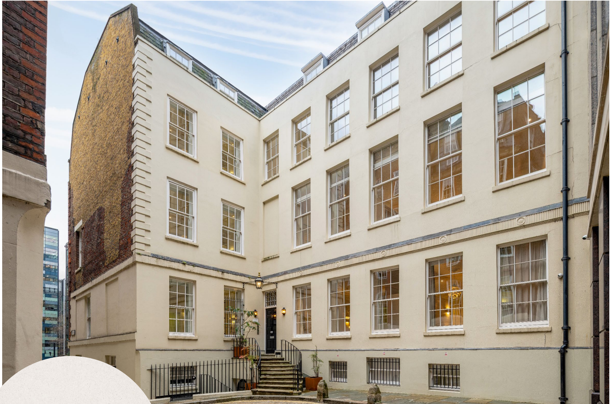
2 SUFFOLK LANE Entrance
