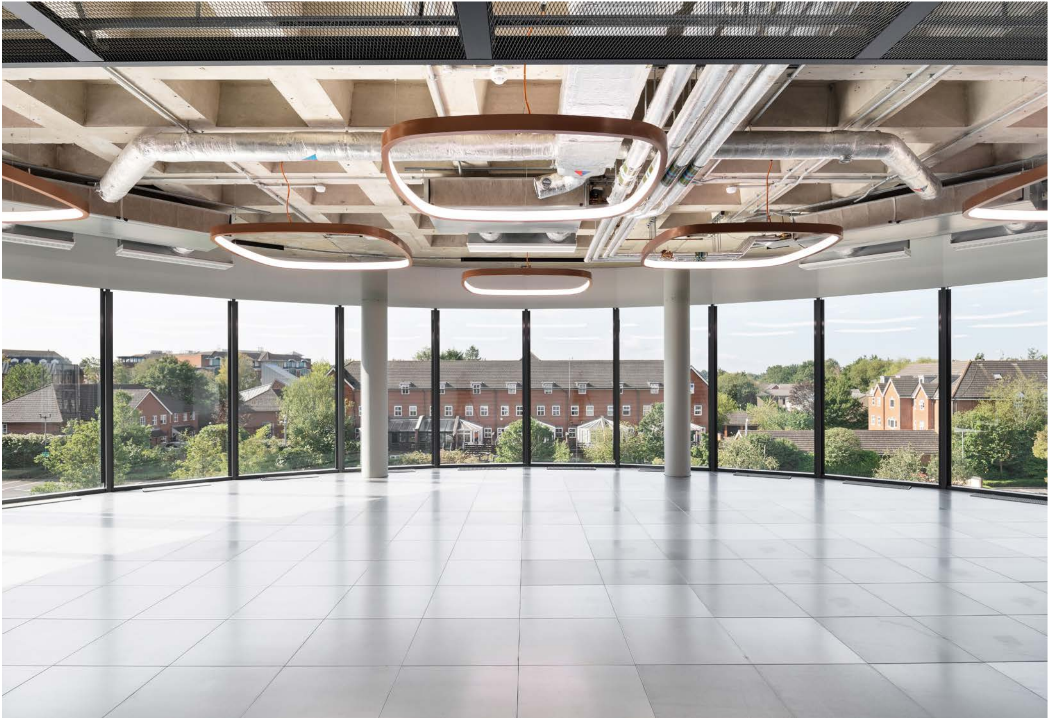
SECOND FLOOR OFFICE
