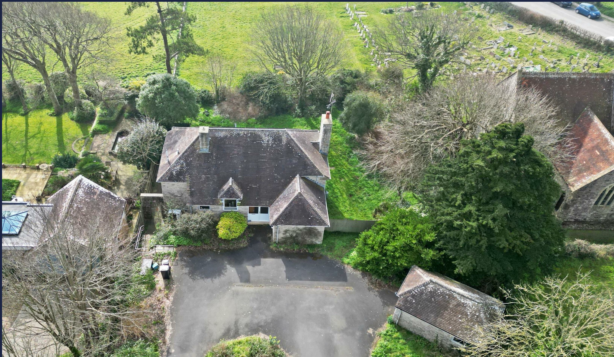
The Rectory, West Road, Wareham
