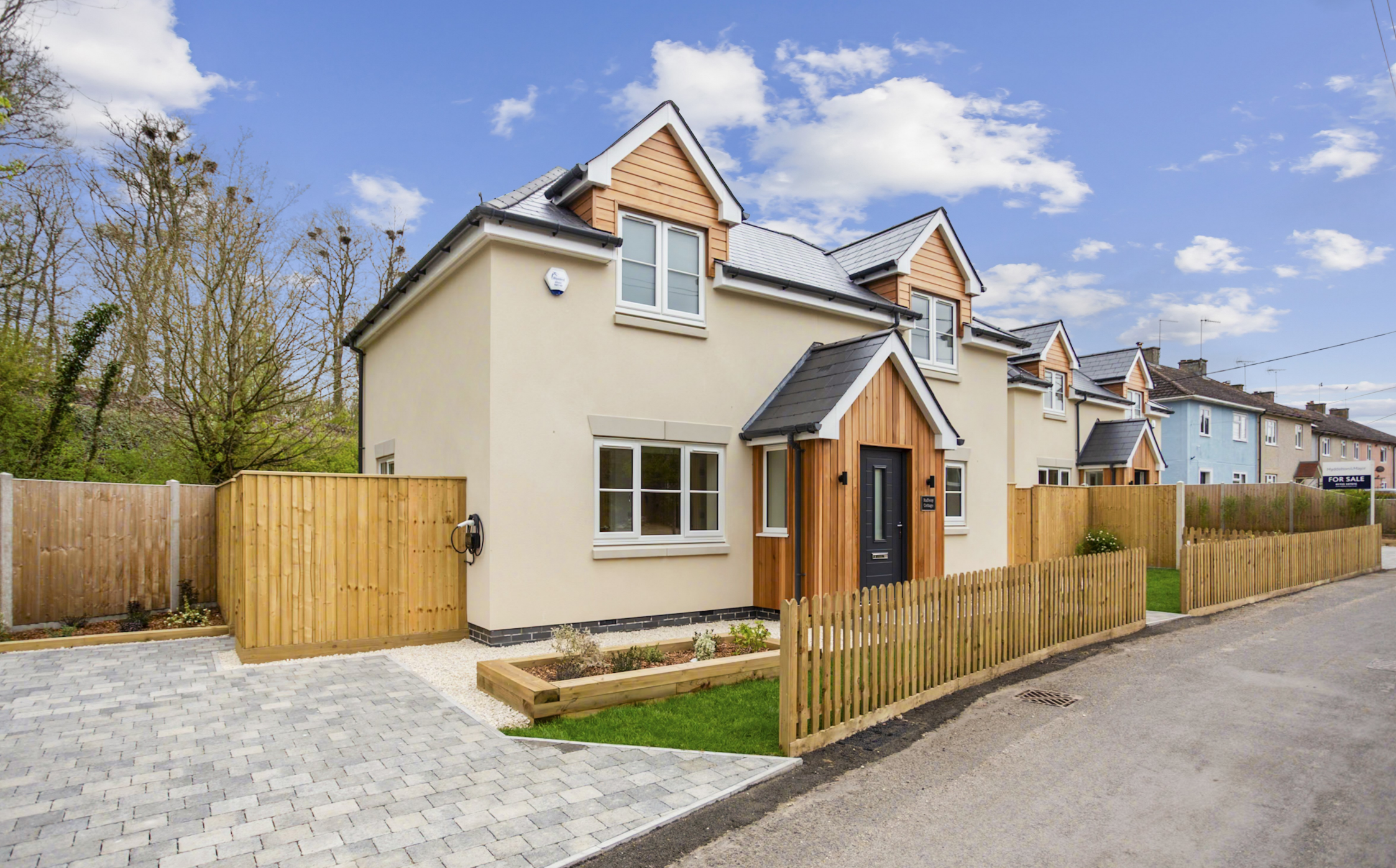
Railway Cottage, Chapel Hill, West Grimstead
