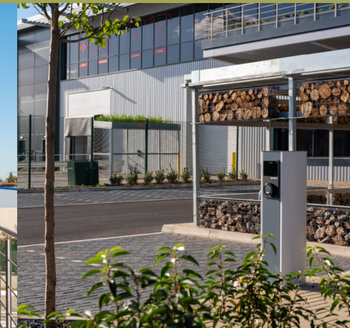
EV point and cycle shelter at SEGRO Park Tottenham
