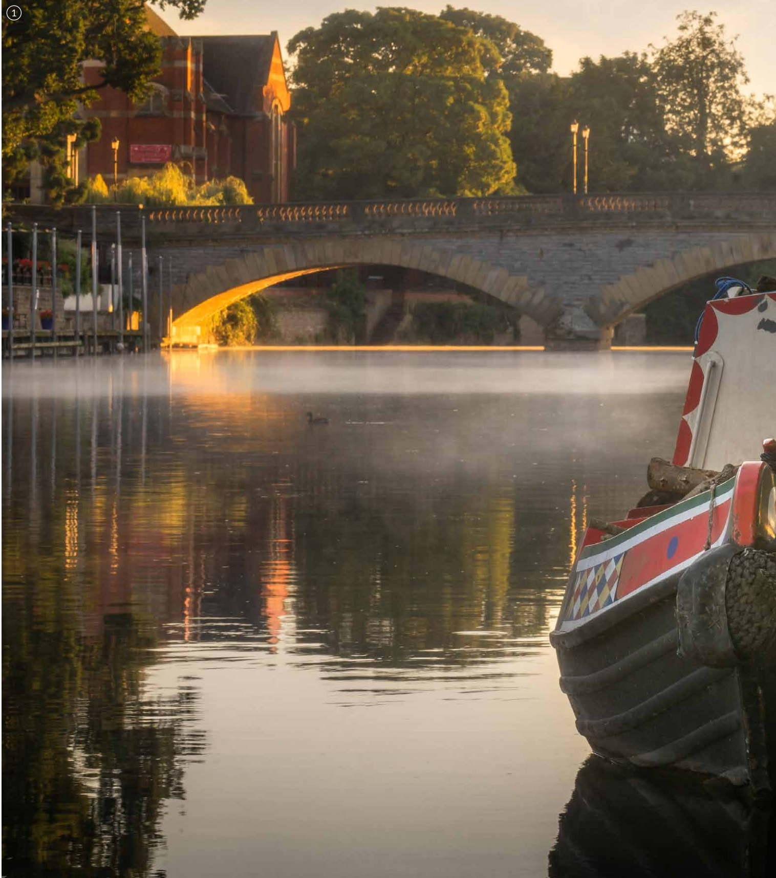
① → Workman Bridge, River Avon
