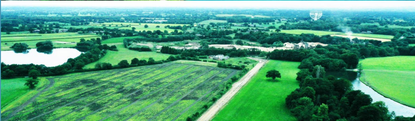
*Waterlines inserted to show prospective outlook upon completion of remediation.
