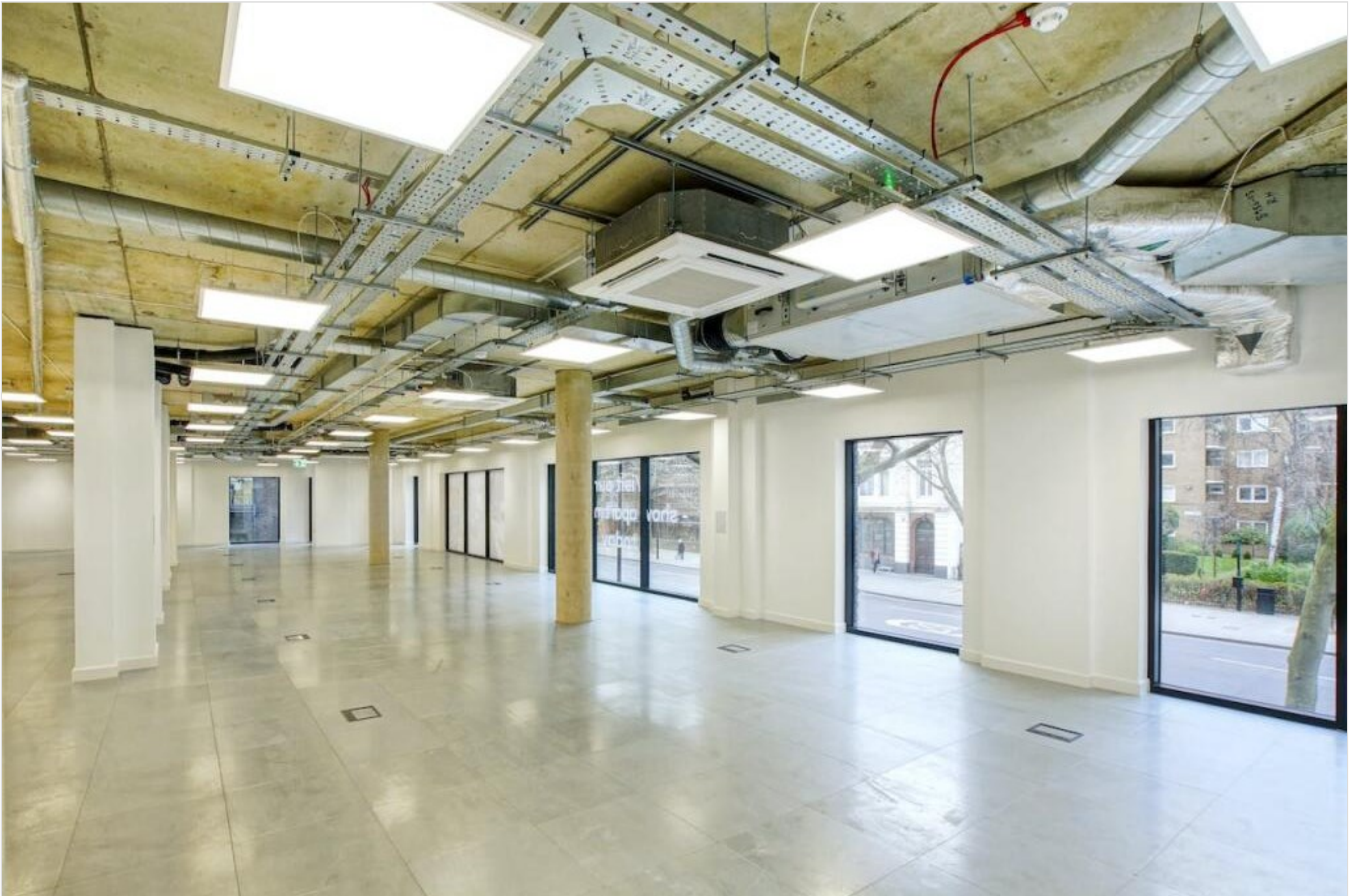
Office 2, The Boulevard, 34 Ufford Street, London, SE1 8QD
