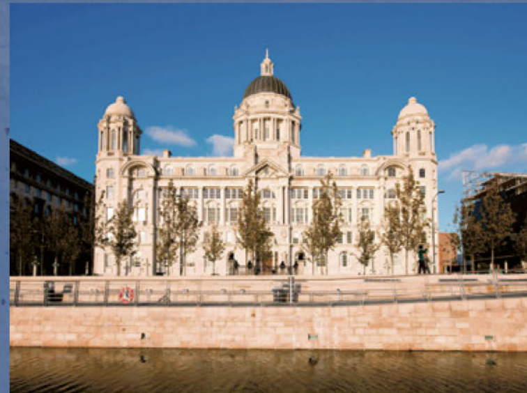
The Port of Liverpool Building – the first of Liverpool's Three Graces. Grade 2 star listed building. Largest, private, completed refurbishment.
