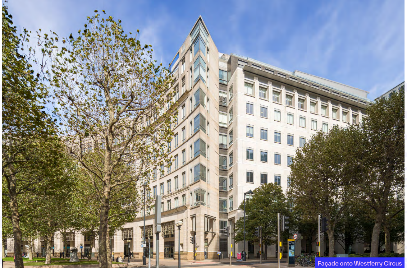
Façade onto Westferry Circus
