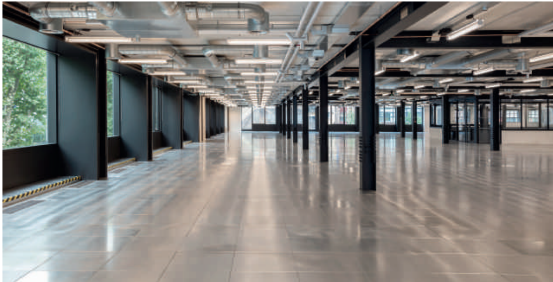
The third floor is delivered to CAT A specification.
