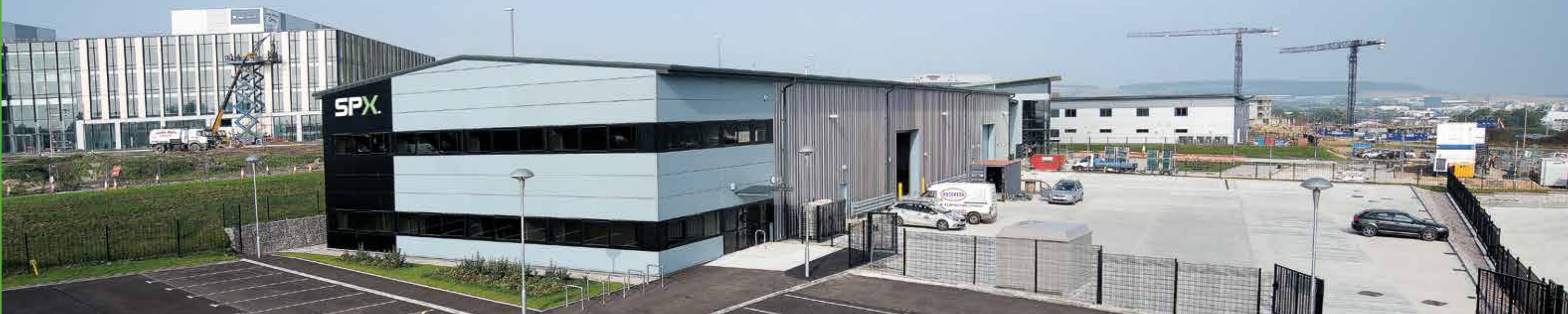
OFFICE AND WAREHOUSE 3 INTERNATIONAL VIEW
