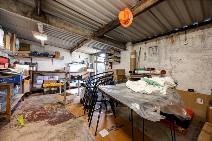
Outbuilding comprising 2 stores, the larger of which (5.91m x 3.55m) has light and power.
