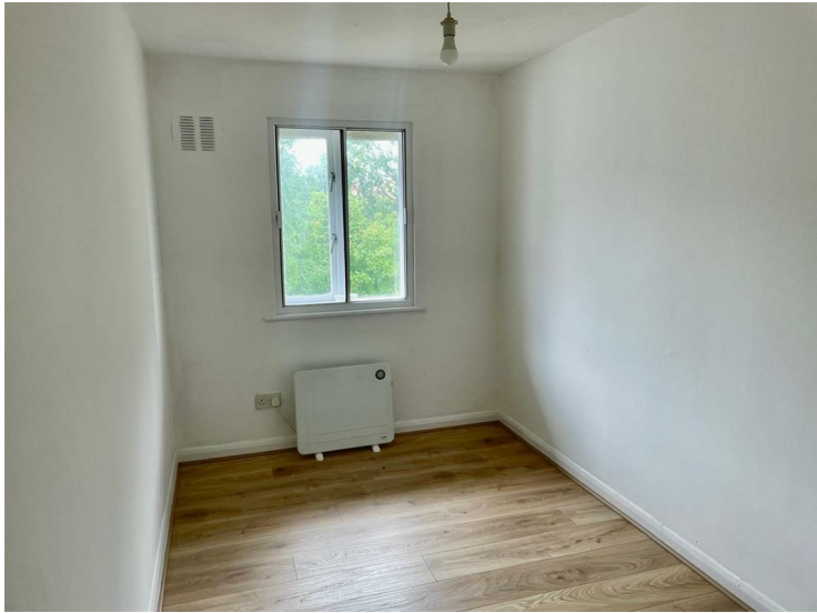
Secondary glazed window, laminate flooring, power point.
