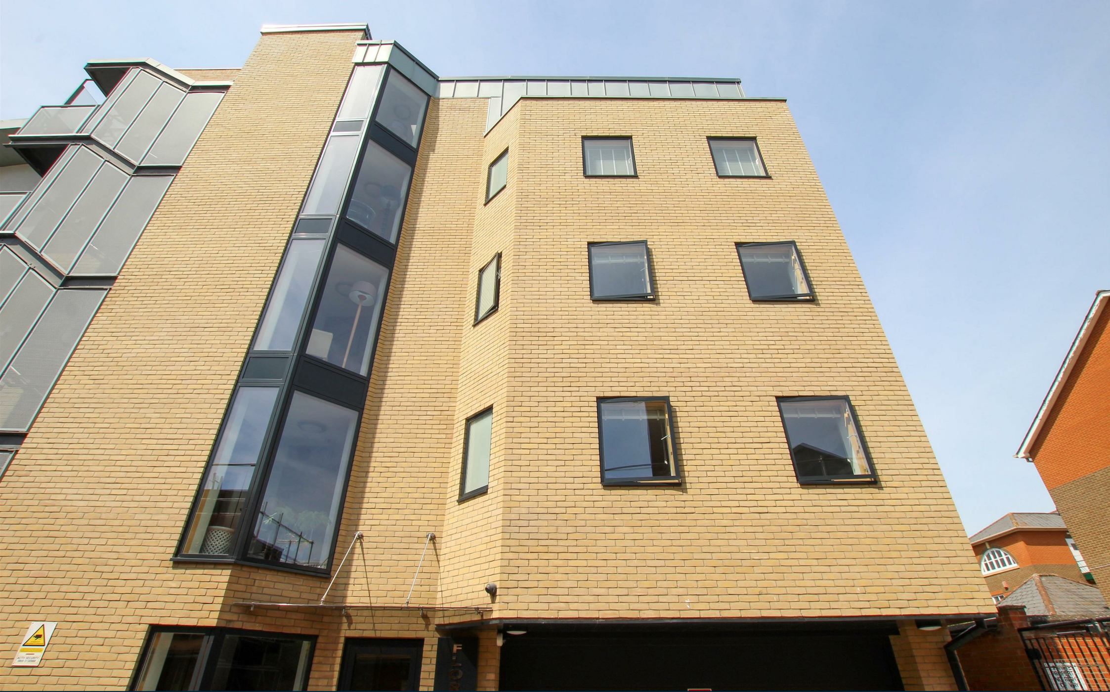
Florian House, Severn Place, Cambridge, CB1 1AQ
