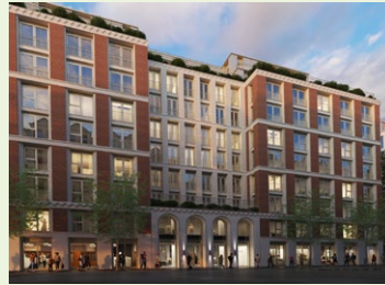
DEAN BRADLEY HOUSE SW1
