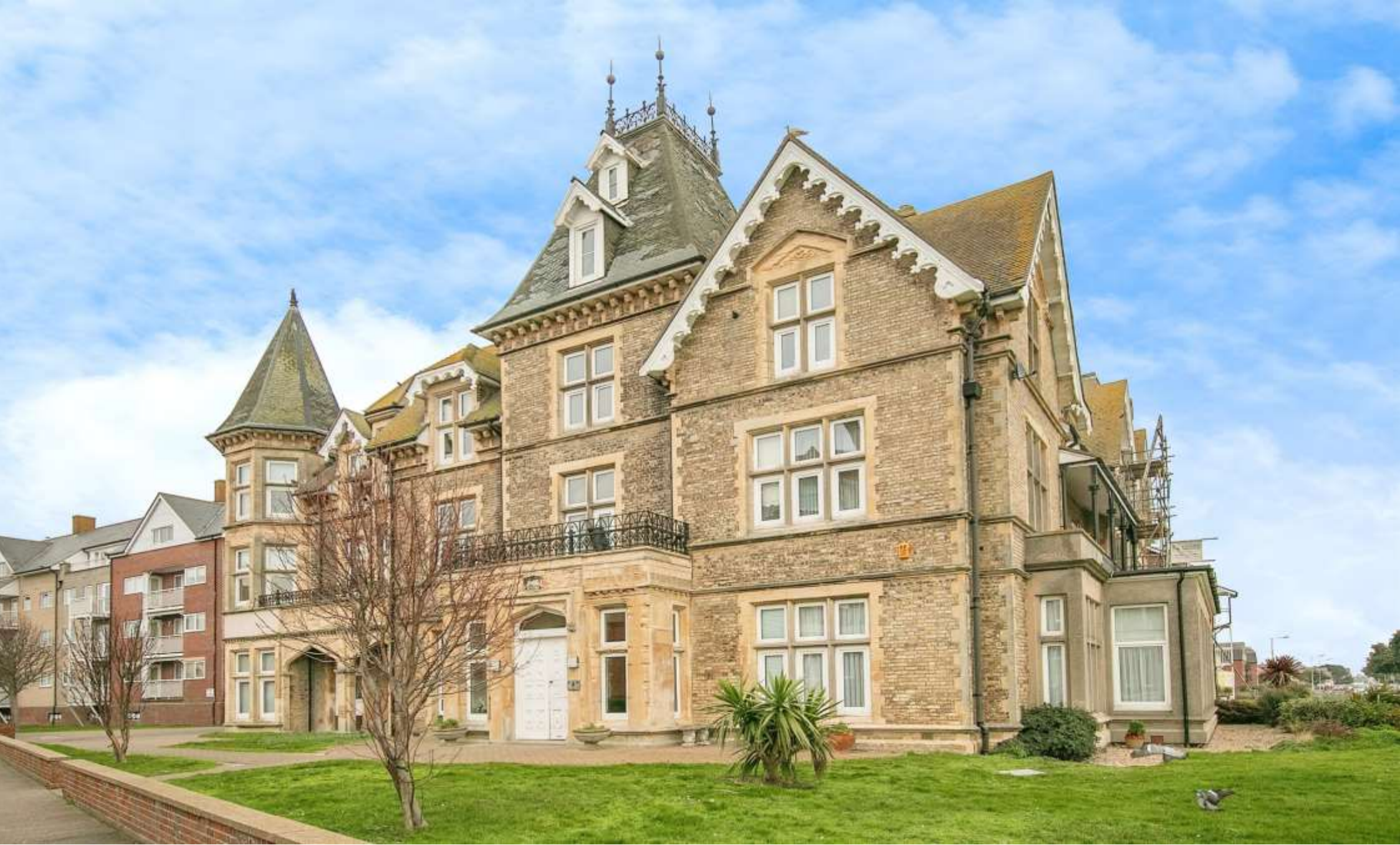
The Towers Vista Road, Clacton-On-Sea CO15 6BY
