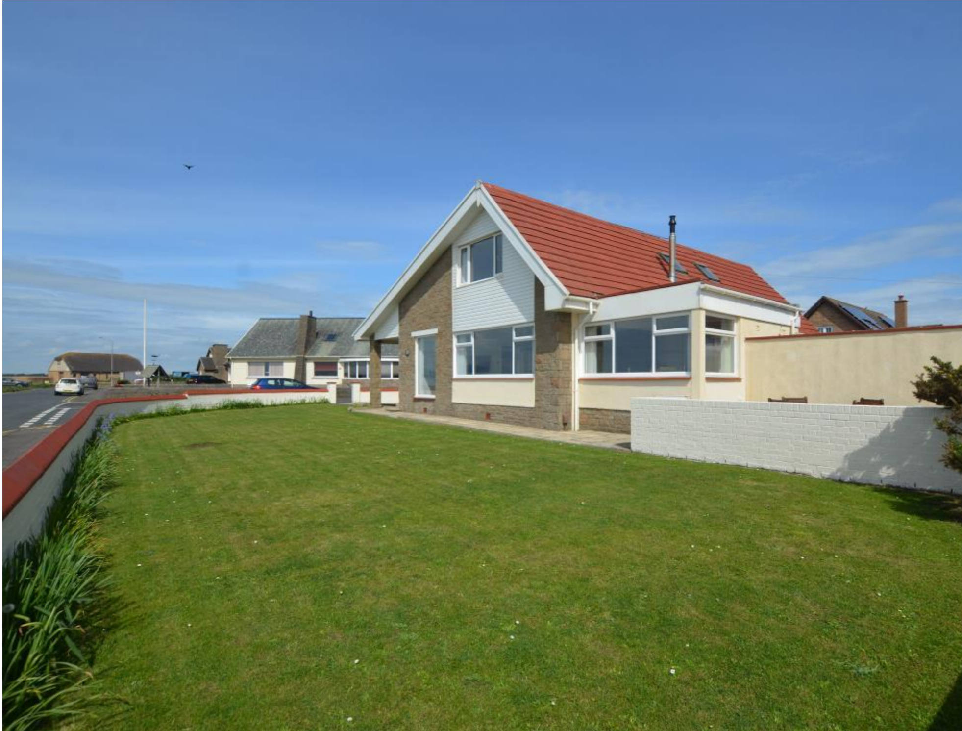
Below: Front Garden and Driveway
