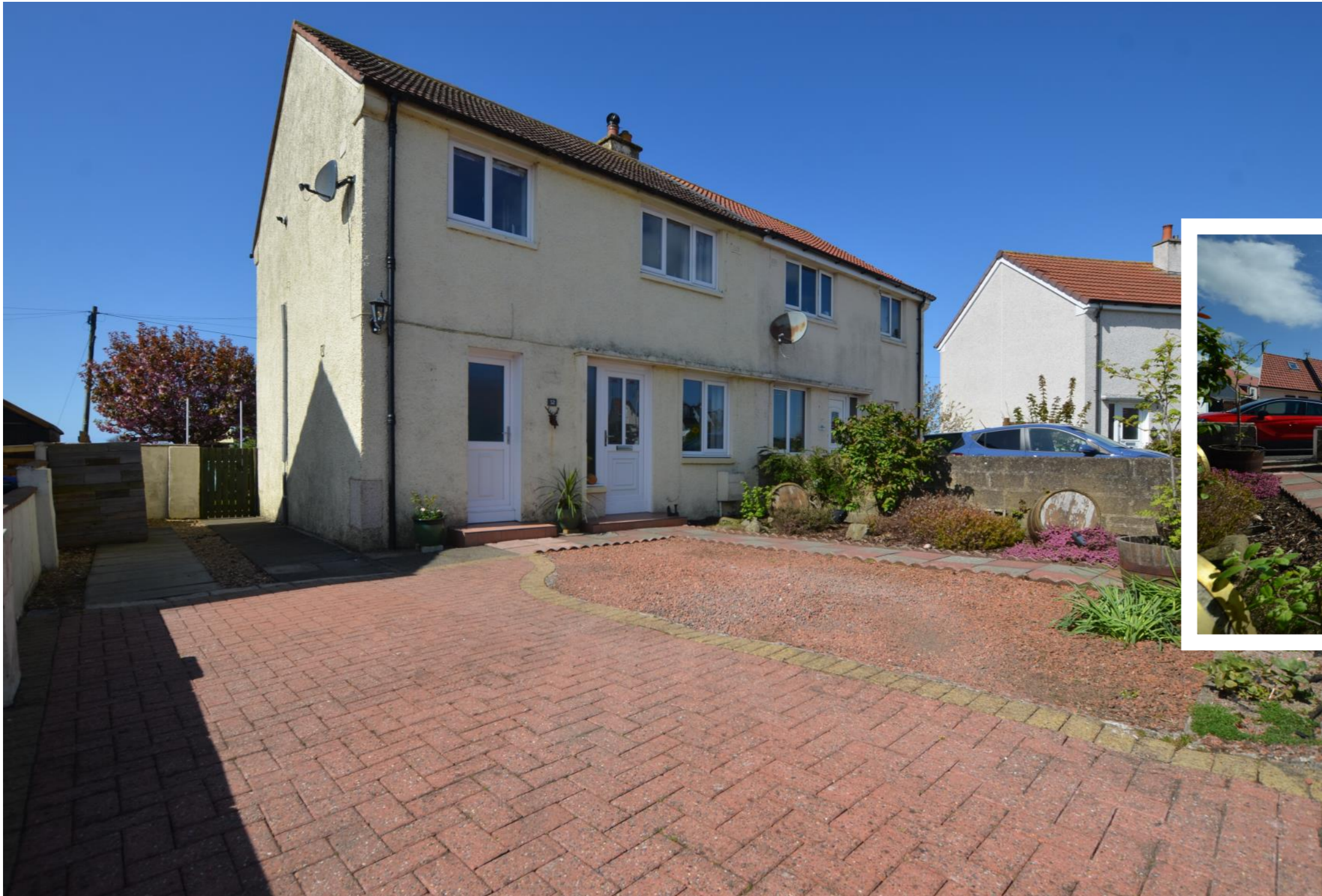
Below: Front of Property
