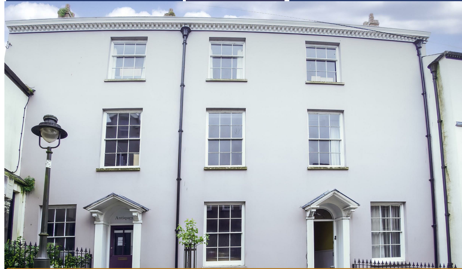
3-4 St. Marys Street, Carmarthen, Carmarthenshire, SA31 1TN
