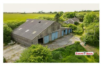
To the one side of the dwelling, there is a large (approx 5,846 sq ft) Atcost type building of steel framed and concrete block construction under pitched corrugated roof. This building comprises a large open plan central section, with LEAN-TOs either side. NB: The roof to a section of a separate LEAN TO has suffered storm damage but the concrete walls seem to be in good condition.
