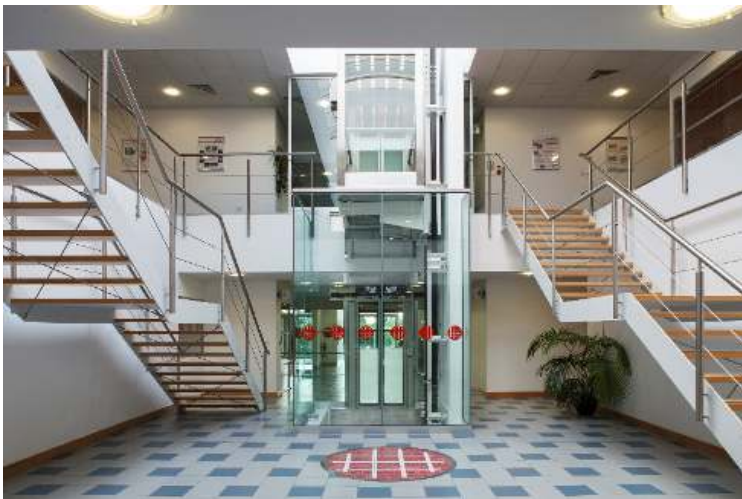
Atrium with Glass Wallclimber Lift
