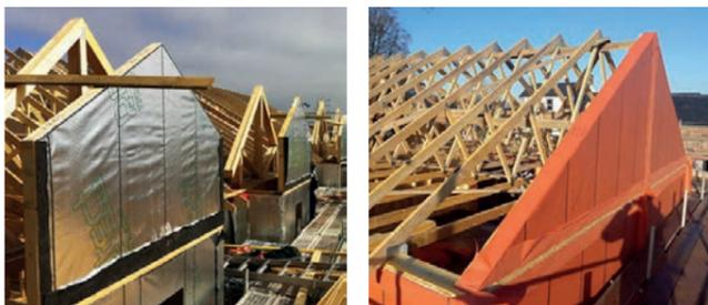
The outer leaf is either brick or block and render depending upon the design. The inner leaf is timber framed incorporating 120mm of insulation with 150mm insulation within the floor construction and 450mm of quilt insulation in the roof space. Our timber framed modern homes have a lower embodied carbon footprint than a masonry built equivalent.
