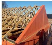
The outer leaf is either brick or block and render depending upon the design. The inner leaf is timber framed incorporating 120mm of insulation with 150mm insulation within the floor construction and 450mm of quilt insulation in the roof space. Our timber framed modern homes have a lower embodied carbon footprint than a masonry built equivalent.
