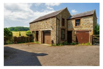
Detached barn with two rooms and space above (accessed via a ladder) and a further store to the side and wood store. Slate roof, stone floors and brick and stone walls.
