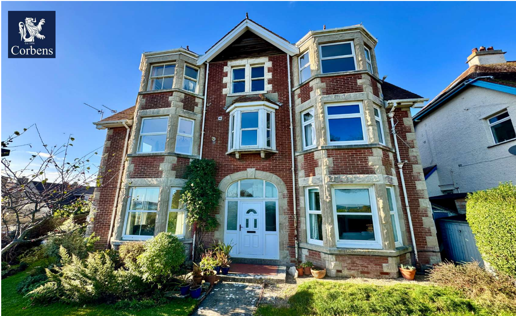
FLAT 2 BAY LODGE, DE MOULHAM ROAD, SWANAGE £240,000 Shared Freehold
