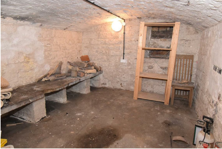
Useful storage space with a vaulted ceiling.
