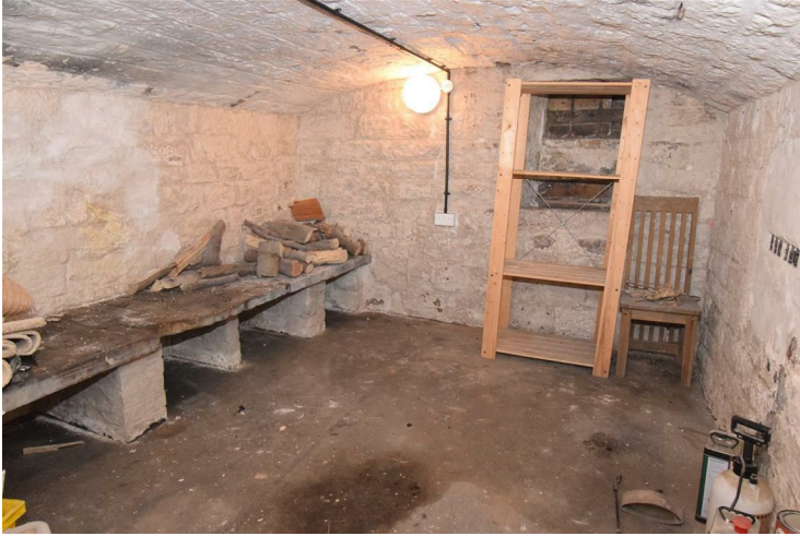
Useful storage space with a vaulted ceiling.
