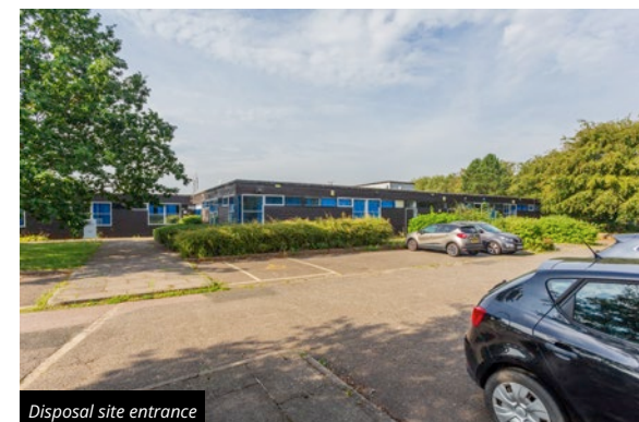
Disposal site entrance
