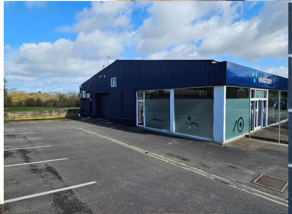
WESTERN VIEW OF BUILDING
