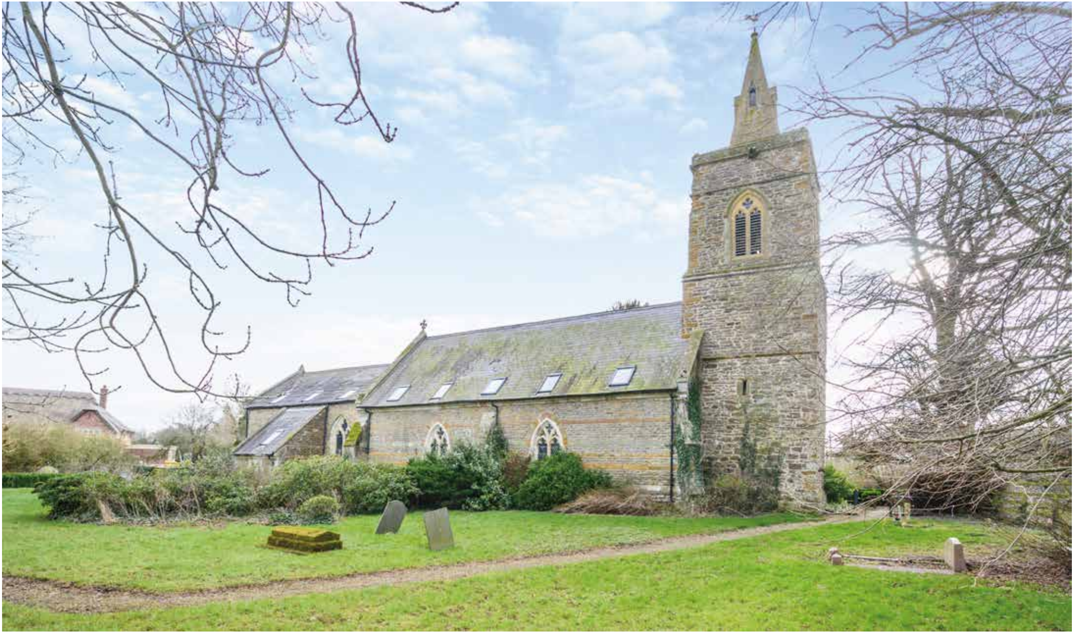
St. Andrews Church Clay Coton | Northampton | Northamptonshire | NN6 6JU
