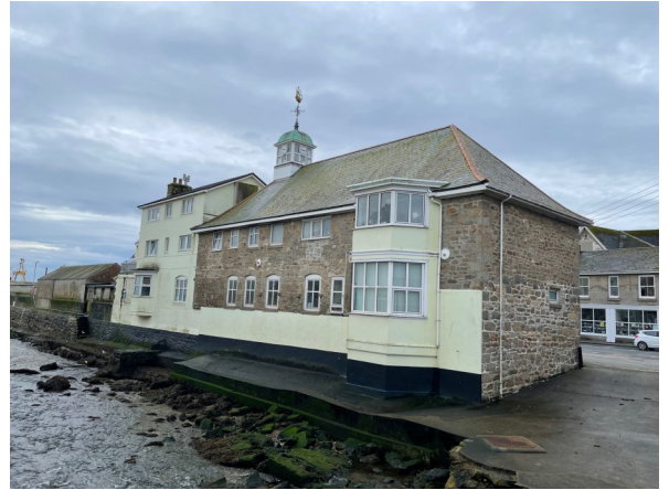
External Elevation Rear
