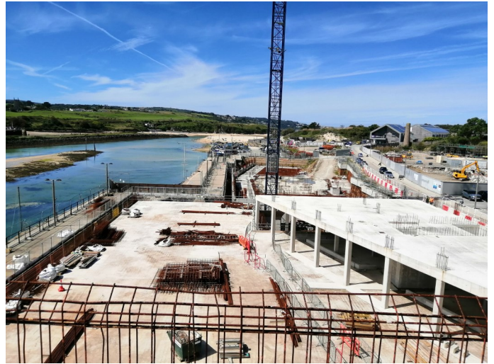
North Quay Square view from B Block
