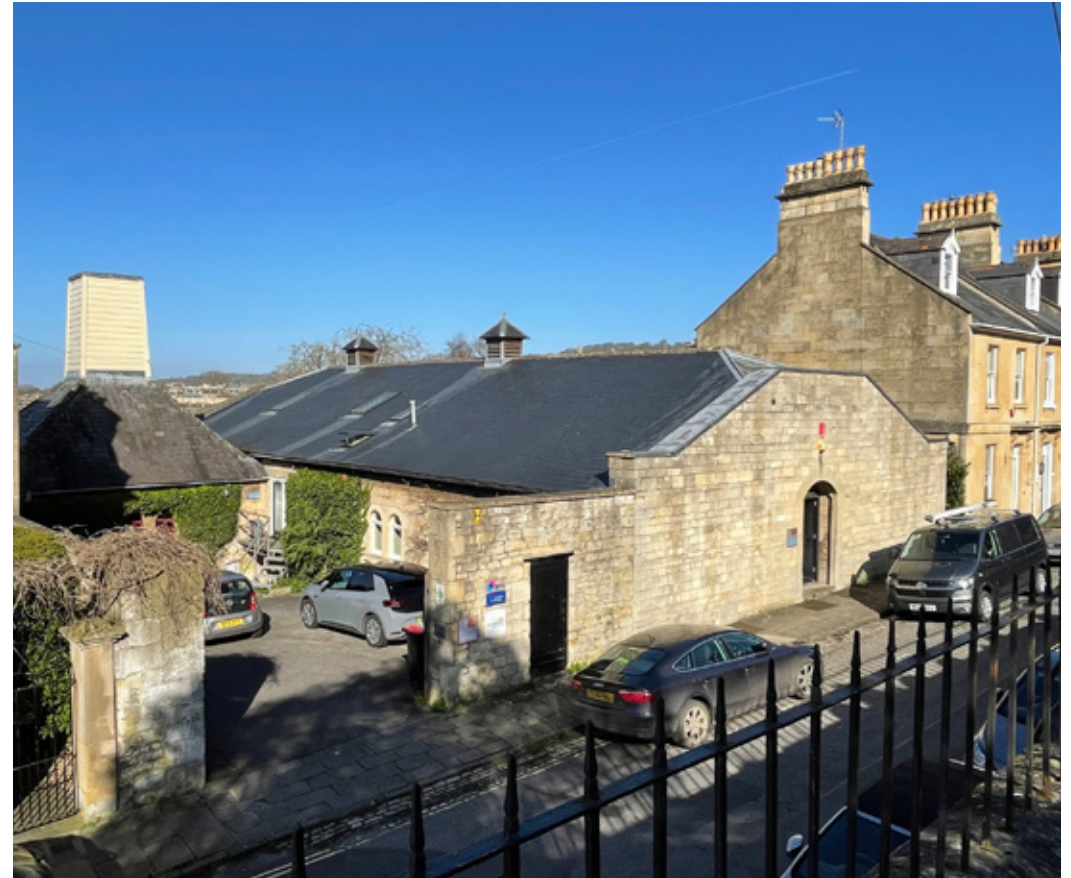
Photograph of rear of building (not forming part of the demise)
